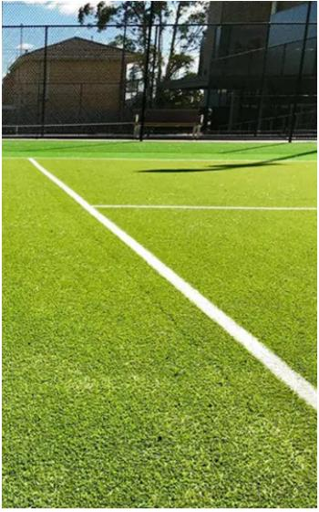
When first installed the artificial grass surface requires a 'settling in' or 'playing in' period where the courts are played on to settle the sand. This ensures optimal distribution of the infill material where the sand settles just below the top of the yarn blade (approx. 1-2mm), and this level should be maintained for the life of the court. Some topping up with sand may be required over the lifespan of the surface.
