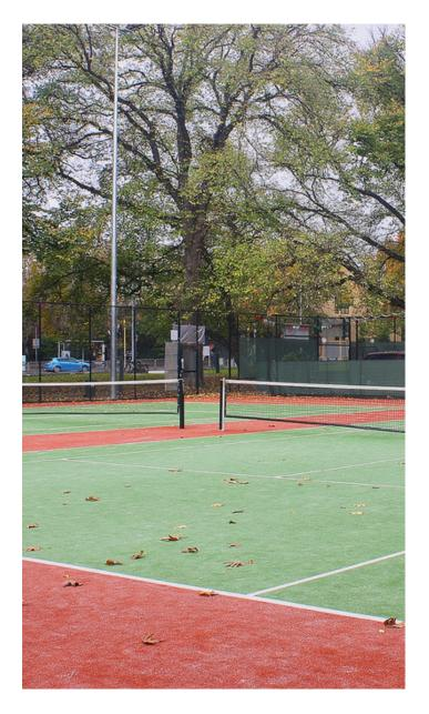
The aim of grooming is to keep the artificial grass fibre 'blades' free and open, and to keep the sand infill evenly distributed. Doing this will enhance surface performance and improve drainage through the grass. If contaminants are not regularly removed, they will be ground into the artificial grass profile and result in contamination of the sand infill, with compaction of the sand and moss/algae growth causing the grass to lose its porosity and premature surface wear.
