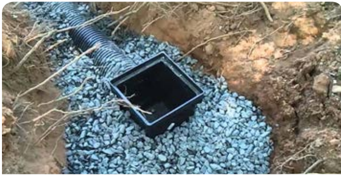
Subsoil Drainage Installation and backfill
