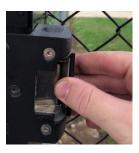
If the electronic strike is working as expected, there may be an issue with the gate. It is common that fencing and gates can move over time, causing locks to become misaligned and not allowing the gate to close correctly. If this is the case with your gate, you will need to investigate with a local fencing/gate contractor, or someone handy from the club to see if you can make changes to the gate/fencing to re-align and help the gate close correctly.
